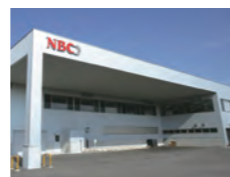
Shizuoka Kikugawa Factory
